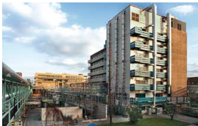
Pilot plant building B 310 (fluids)
