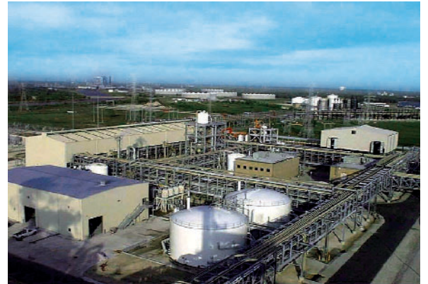
Chlorine electrolysis plant, Baytown, USA
