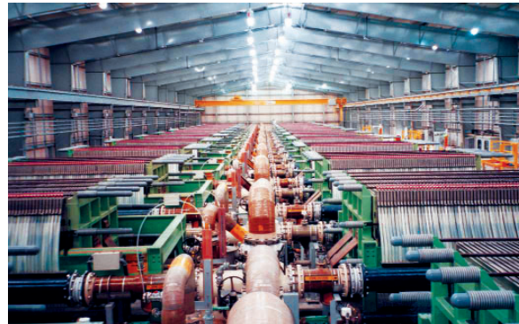
Cell room, Baytown, USA
