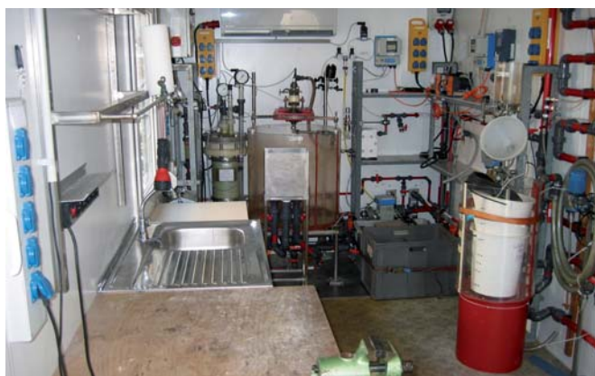
Mobile Lab Container for pilot tests on site
