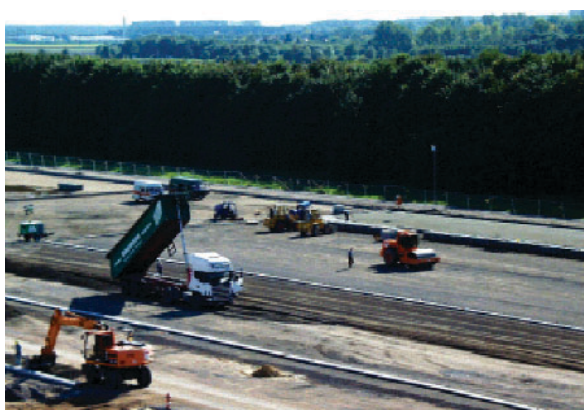
Ground surfacing for a logistics center
