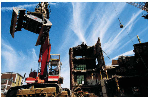
Demolition of production buildings
