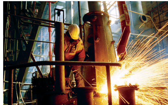
Dismantling of reaction vessels in a chemical plant
