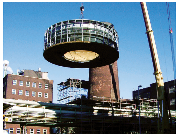
Demolition of a water tower in the Leverkusen Chemical Park
