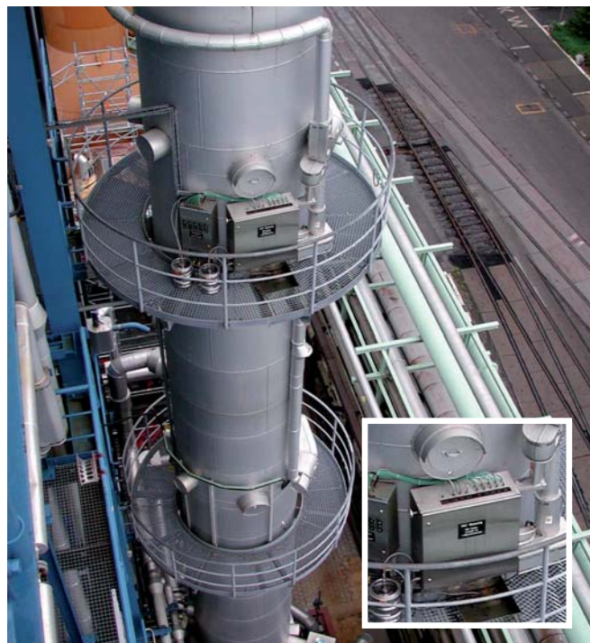
Online NIR measuring point on a distillation column
