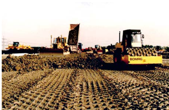
Installation of a mineral sealing layer (landfill construction)
