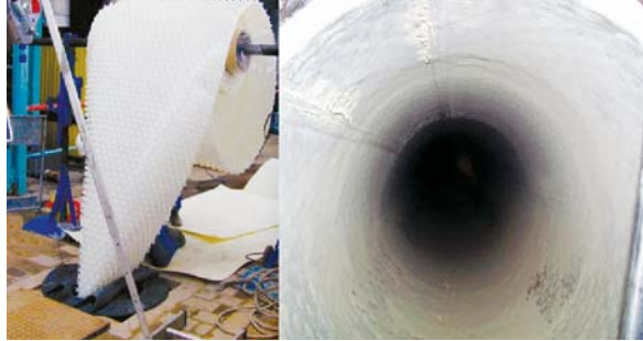
Pipeline renewal through Trolining®
