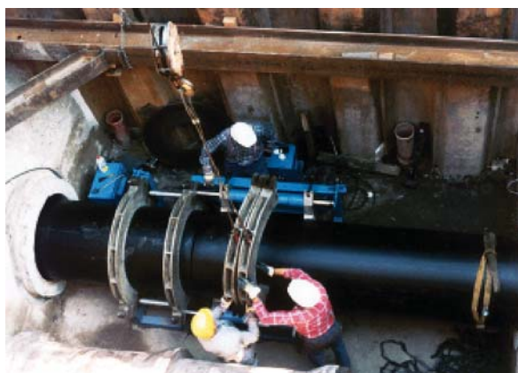
Relining of PE pipes using pre-welded sections
