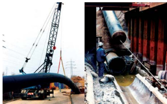
Relining using endless pipe, insertion above ground
