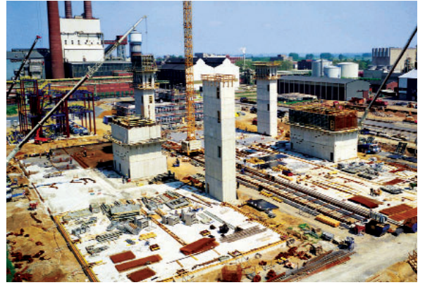
Construction of a production complex in Dormagen
