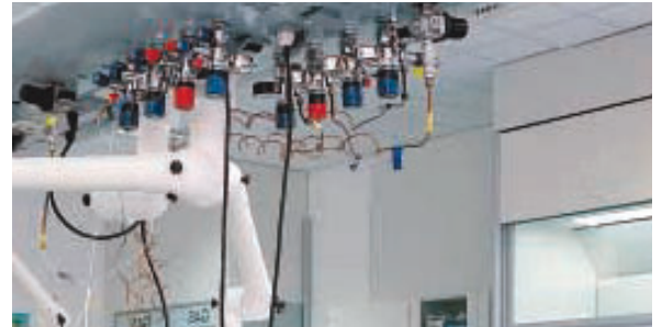
Innovative solutions, e.g., for the supply and removal of media from above the workplace
