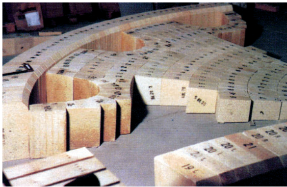
Preparations for lining work on a sewage sludge incineration plant
